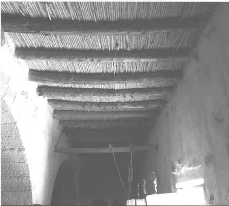
This reconstructed house in the Nazareth Village in Israel shows a roof like one of the four friends could have broken through to bring their paralyzed friend to Jesus (Luke 5:19).
